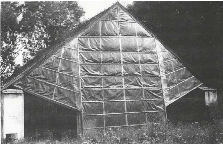
Figure 8. A wall collector for drying agricultural products
